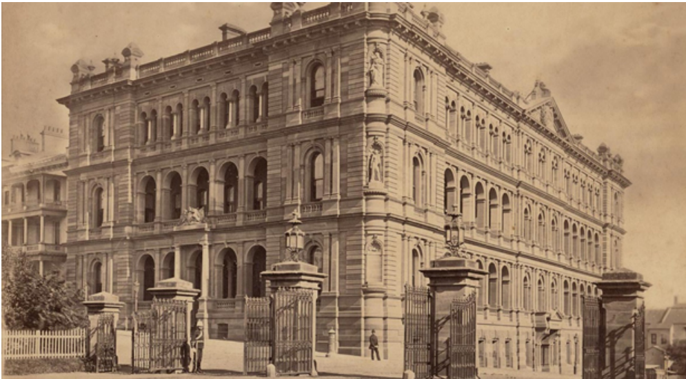
Colonial Secretary's Building on the corner of Macquarie and Bridge streets, headquarters of the Aborigines Welfare Board (Mitchell Library, State Library of NSW - SPF / 248)
